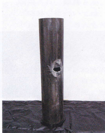
●鋼管柱施工前
